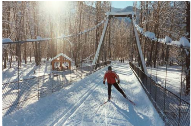
The Suspension Bridge Near Mazama, WA.
